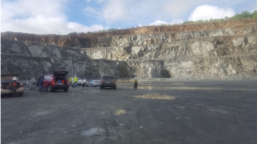
The pit at Garrisonville
